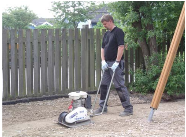
Compact the subbase
