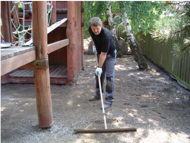
Level out the subbase material
