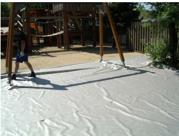
Place the geotextile fabric in top of the prepared subbase and install the ErgoPlay rubber tiles
