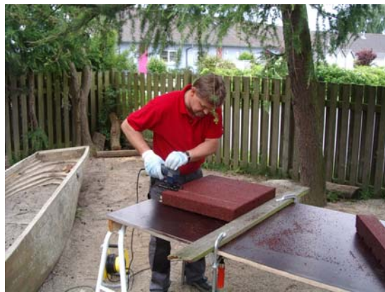
Cutting can be done by the use of e.g. a heavy-duty carpet knife or a sabre saw
