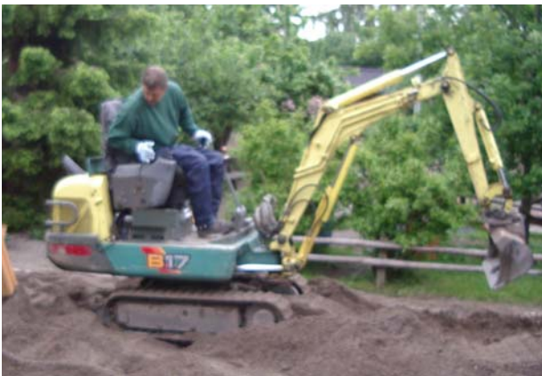
Removal of topsoil
