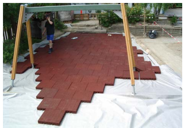
Place the geotextile fabric in top of the prepared subbase and install the ErgoPlay rubber tiles
