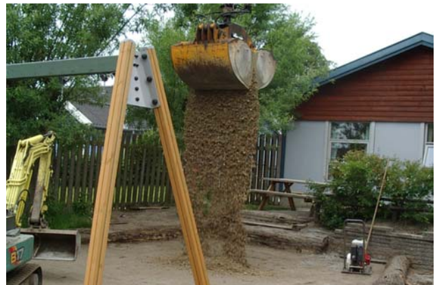
Add the subbase material
